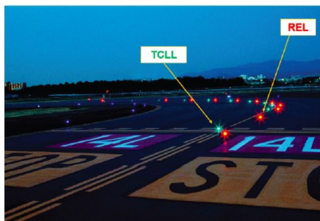
Figure 3 Illuminated Runway Entrance Lights (RELs) (Source: JCAB)
