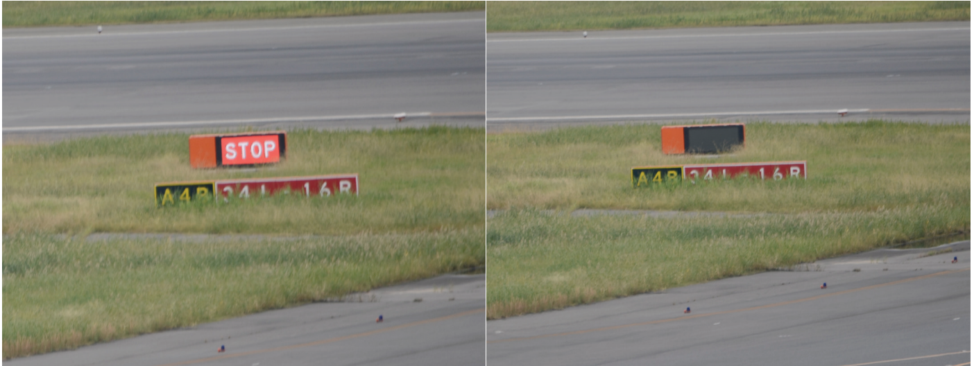
Figure 1: On left, Variable Message Sign displays "Stop". On right, Variable Message Sign off.
