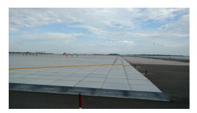
Figure 3 EMAS installation on Boston Logan Departure End of 15R. Photo Courtesy of Mark Crystal.
