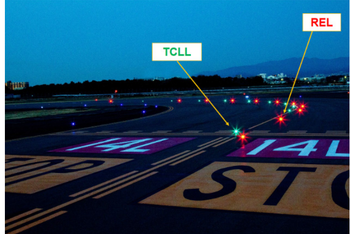
Figure 3 Illuminated Runway Entrance Lights (RELs) (Source: JCAB)
