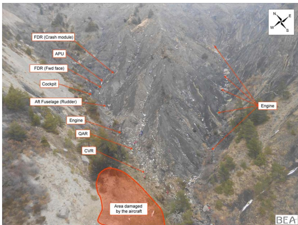
Figure 12 - general view of the accident site
